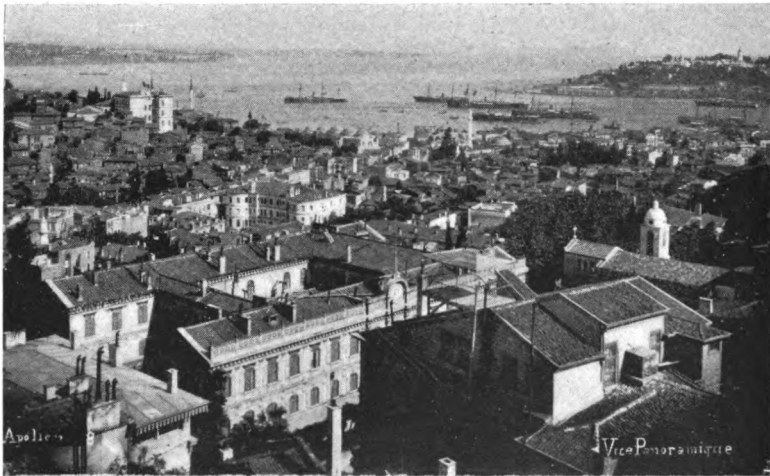
VIEW FROM RED CROSS HEADQUARTERS, SHOWING GOLDEN HORN, BOSPHORUS AND MARMARA.
